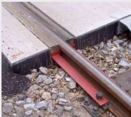
Installation in slab track
