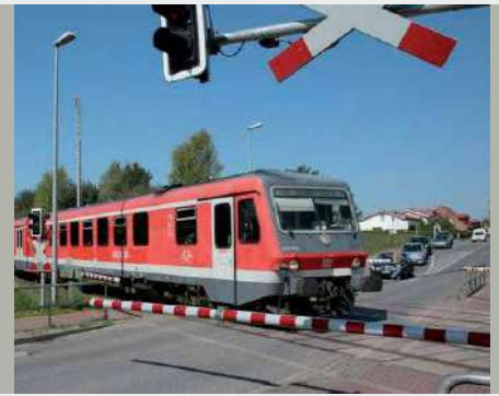
Level crossing with Sylomer® Rail Groove Fillers
