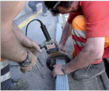
Welding the groove filler profiles together
